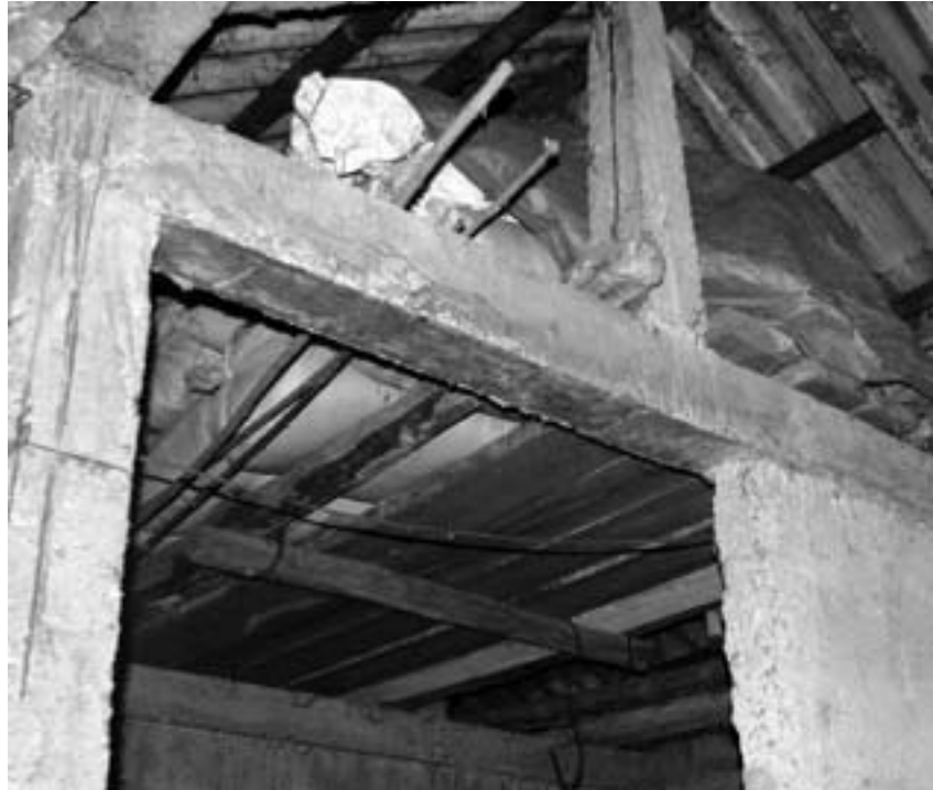
Many households now have platforms for safe storage during the flooding season.
