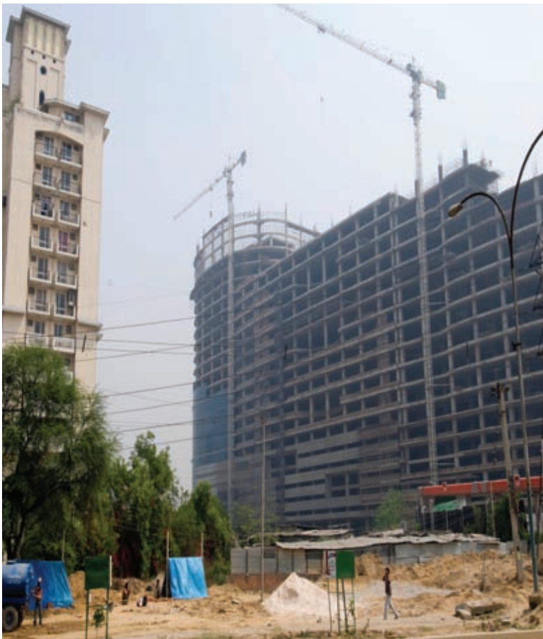
Construction Site, Gurgaon
