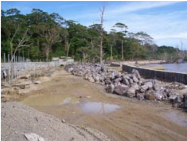
Biodiversity Park, Road being constructed at Chidiyatapu, Andaman Islands
