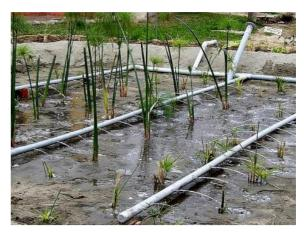
Figure 6. VFB under construction, during influent pumping with greywater to test for uniform distribution in Lima, Peru. Note the small holes in distribution pipes. The entire surface is used as an inlet area, and the pipes are later covered with gravel after completing the testing (photo by H. Hoffmann, 2008).
