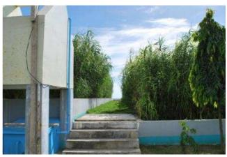
Figure 27. Subsurface flow CW in Bayawan city, Philippines. The path in the middle separates the VFB and the HFB (photo by J. Boorsma, 2009; project supported by GIZ)<sup>24</sup>.
