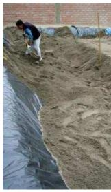
Figure 9. Left: VFB during construction in Palhoça, Santa Catarina, Brazil; drain pipes situated on top of the PE liner are being covered with gravel. Right: VFB in Lima, Peru during filling with sand (photos by H. Hoffmann, 2007).
