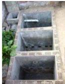
Figure 15. Left: Septic tank schematic. Right: 3-chamber septic tank under construction at a house with 15 habitants in Lima, Peru (sources: H. Hoffmann, 2009).
