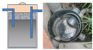
Figure 14. Left: Grease trap schematic. Right: Opened grease trap used for effluent of a kitchen sink of a household in Lima, Peru before wetland treatment. The inner bucket can be taken out to remove the grease (sources: H. Hoffmann, 2010).
