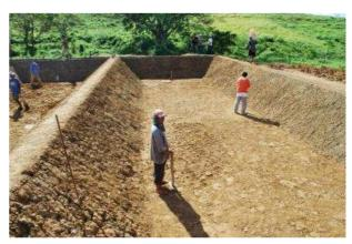
Figure 7. VFB under construction in Bayawan City, Philippines; the wetland will treat wastewater from a landfill (photo by J. Boorsma, 2009; project supported by GIZ).
