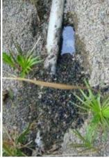
Figure 28. Left: Malfunctioning grease trap with too much sludge accumulation. Right: the sludge from the grease trap obstructs the infiltration area of the CW which has become black because there is no oxygen transport anymore and it has become clogged (photo by H. Hoffmann, 2009).
