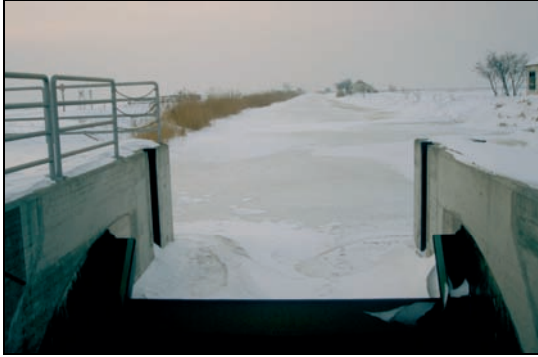
Figure 6.6. Sluice of the Hanság-Channel
