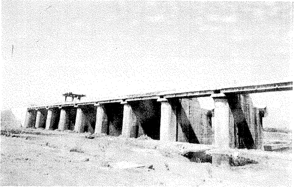
Un-gated bays d/s view on 28.04.2011. Cofferdam in the background
