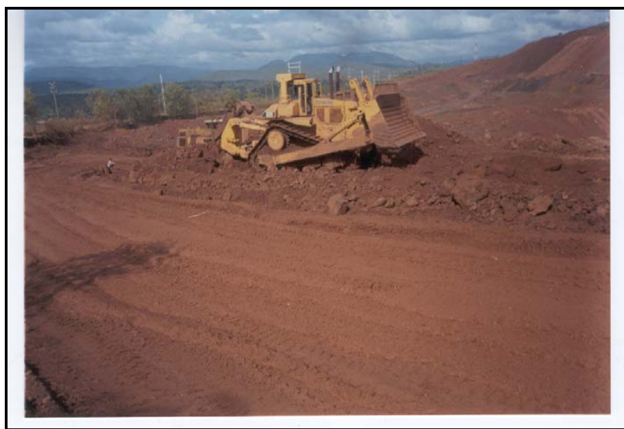
Fig. No. 5.1.2.1 Ripper Dozer Working at Bicholim I/O Mines in Goa
