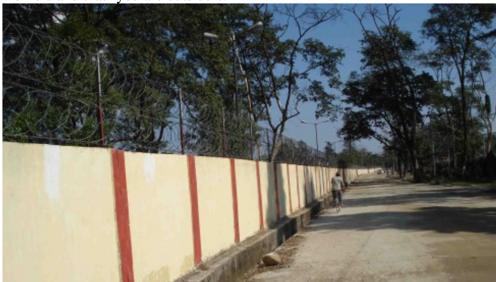
The barbed wire fence enclosing the NHPC complex at the Subansiri dam site.
