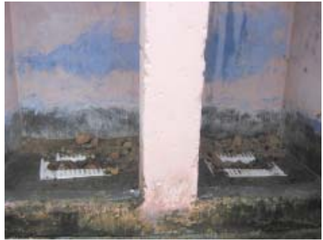
School Toilet in Nalanda
