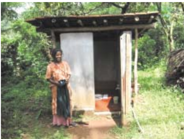
Upgraded toilet in Shimoga
