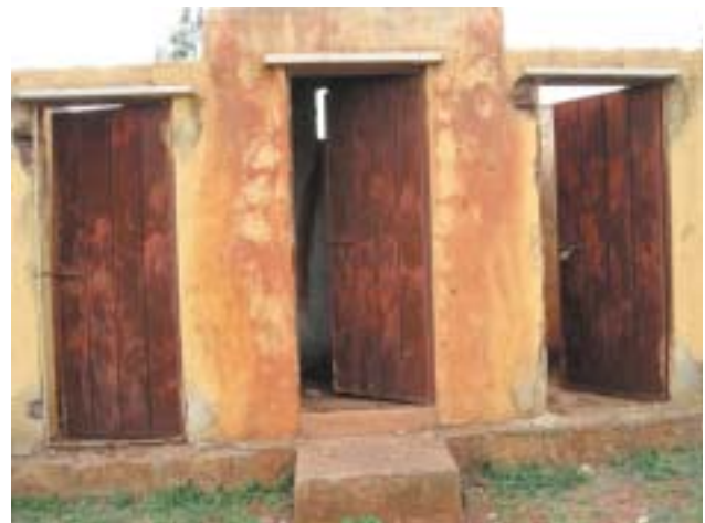
Reconstructed school toilet in Bidar
