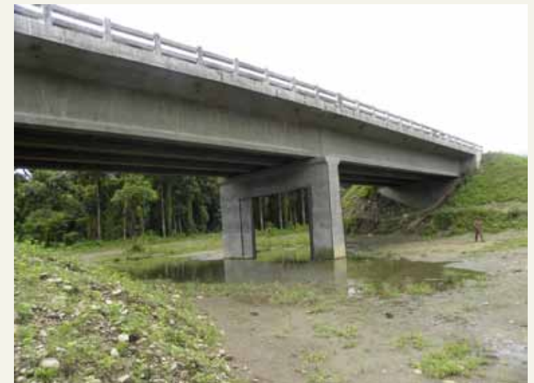
Figure 7 – Elephant underpass in which portal type piers replace wall type thereby providing lateral visibility
