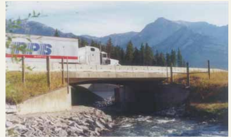
Figure 11 - View of the underpass with side space from a different location
