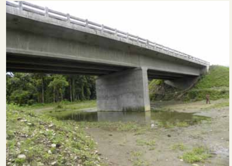
Figure 6 – Elephant underpass with solid wall type pier
