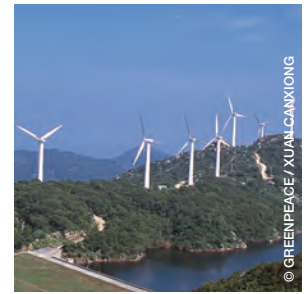
Wind turbines at the Nan wind farm in Nan'ao.
