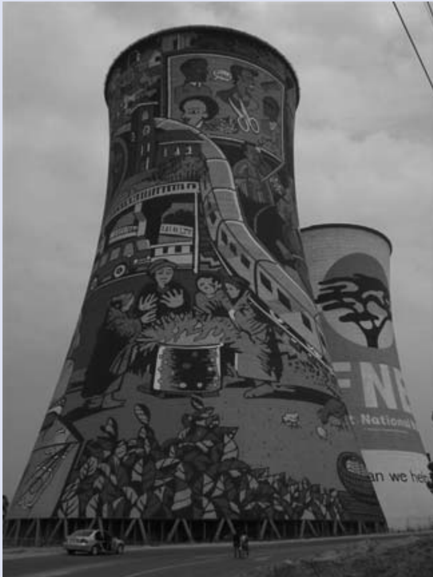
The cooling towers of an old power plant in Soweto are no longer in use. One now depicts local art and the other advertises a local power company, Photo by Schlaeger, reproduced under the terms of the Creative Commons.
