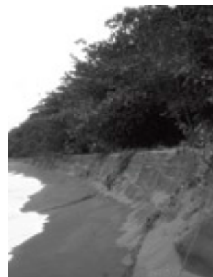
Coastal erosion, Costa Rica Photo courtesy of Sonia Gautreau
