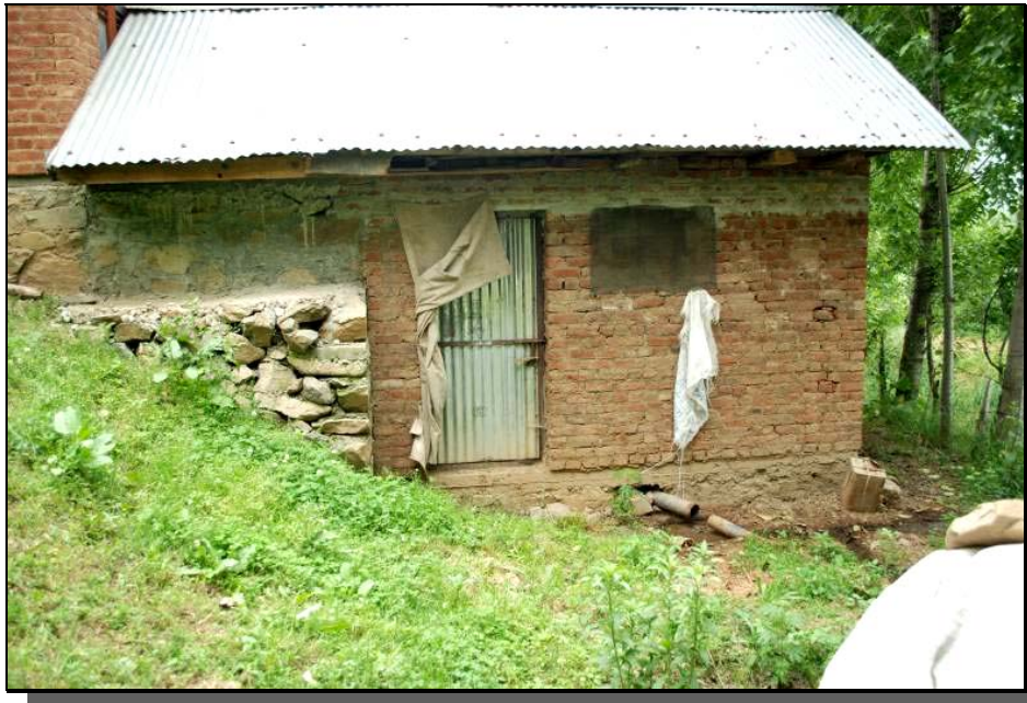
Fig. 34 A picture of a cattle shed in Saidpora village in Central Wildlife Division where the wooden door was replaced with iron door
