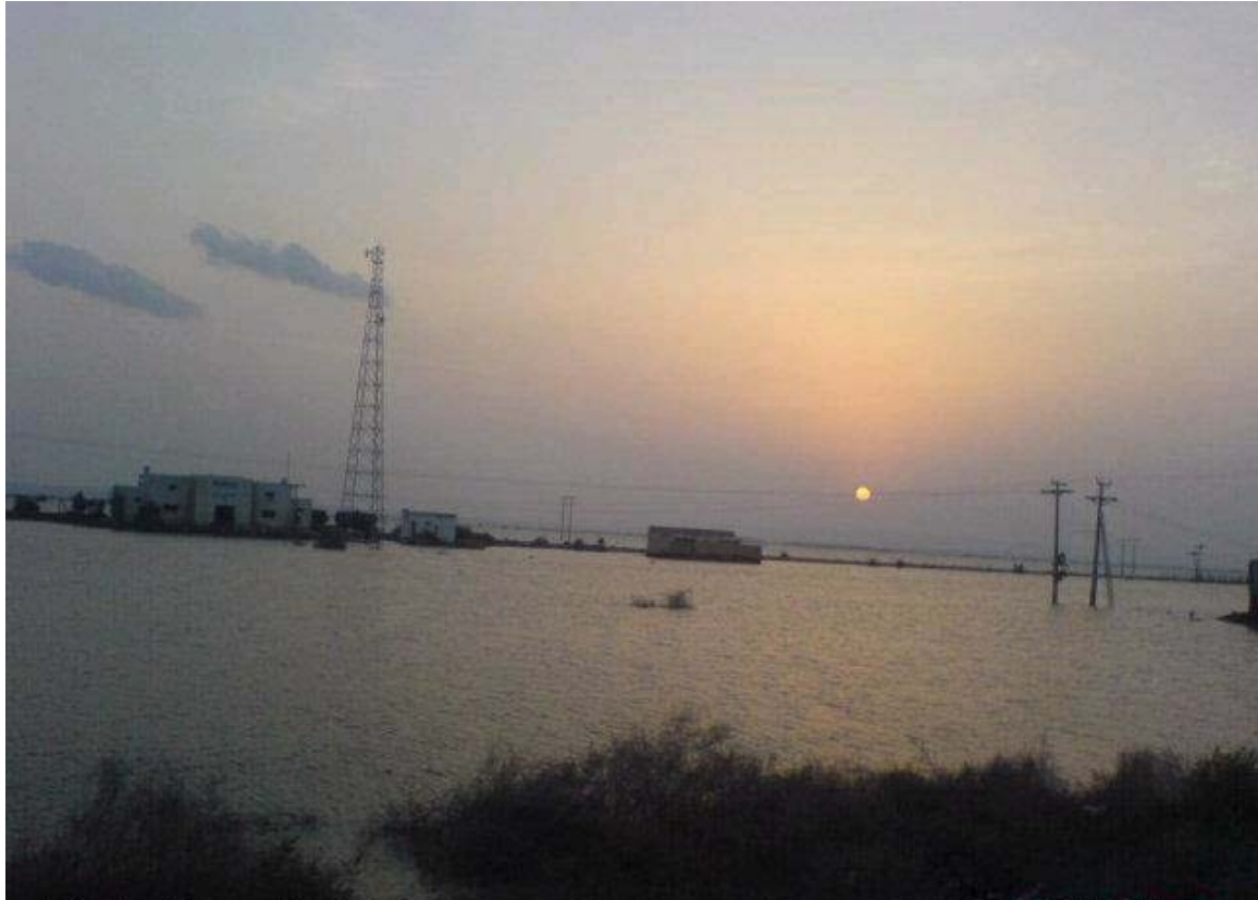
Flooded power station (Copyright: Author)
