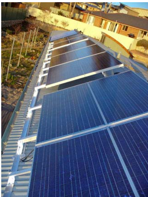
Solar panels (Copyright: Jeff Knowles and DEWHA)
