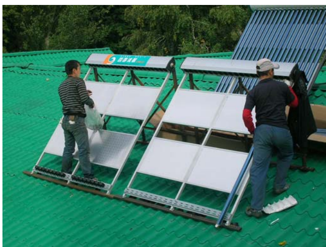
Setting of the solar heating collector (Copyright: A. Nehaenko, PF "EcoIDEA")
