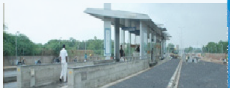
Bus stop under construction in Ahmedabad BRTS
