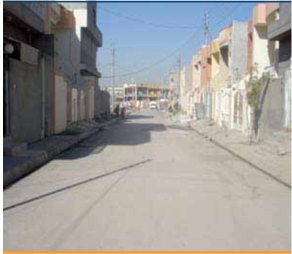
Figure 10.4 Badawa after Completion of Rehabilitation Works
