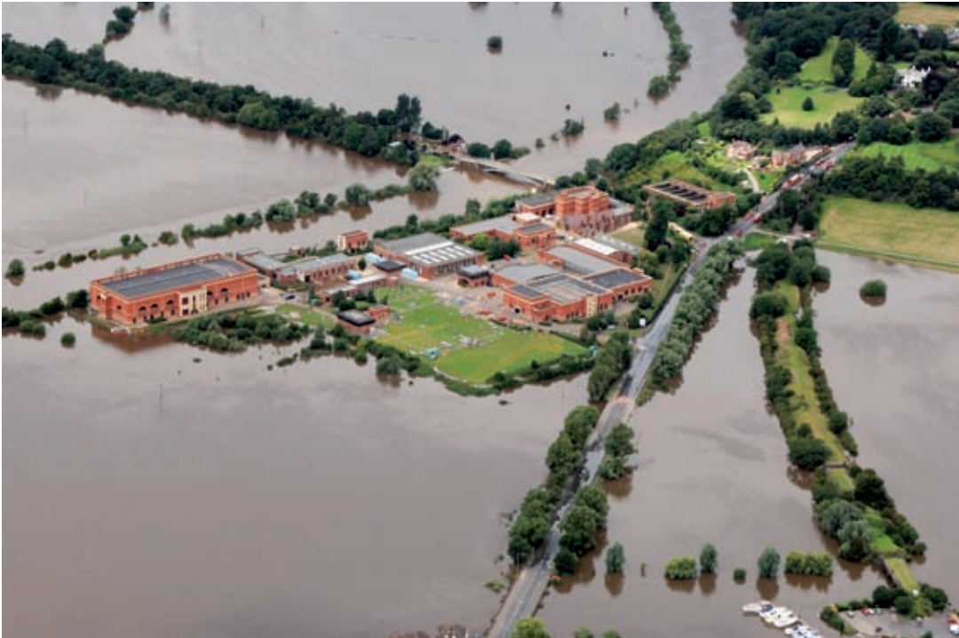
Flooded drinking-water plant, Mythe, Gloucestershire, United Kingdom, 2007
