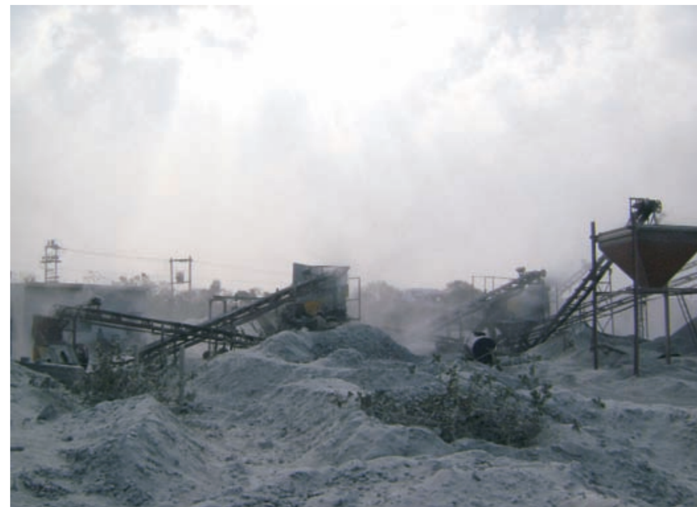
Stone crushing unit needs dust control systems to minimize air pollution
