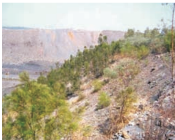
Slope stabilization for soil conservation
