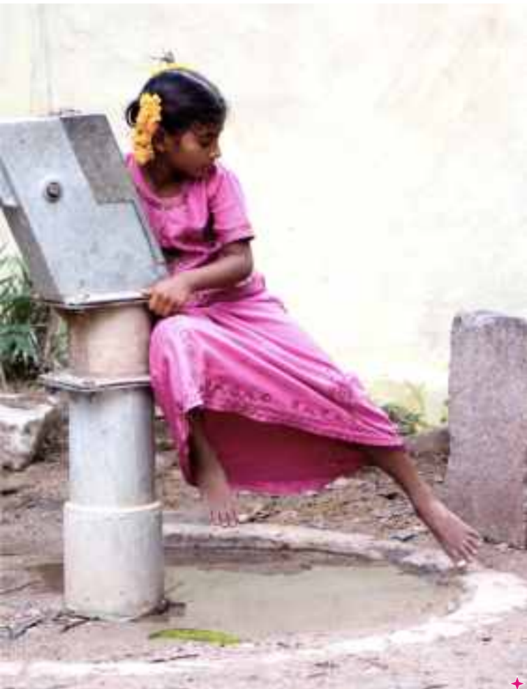
Above handpump repaired, cleaned and freshly lined with bleaching powder.
