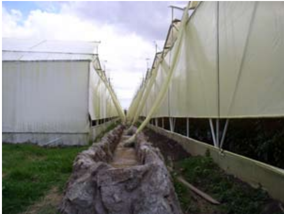
Rainwater harvesting and conveyance in stone and concrete drains
