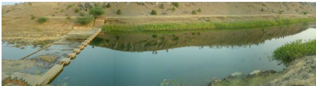
Checkdam in village of Dotad Jhabua
