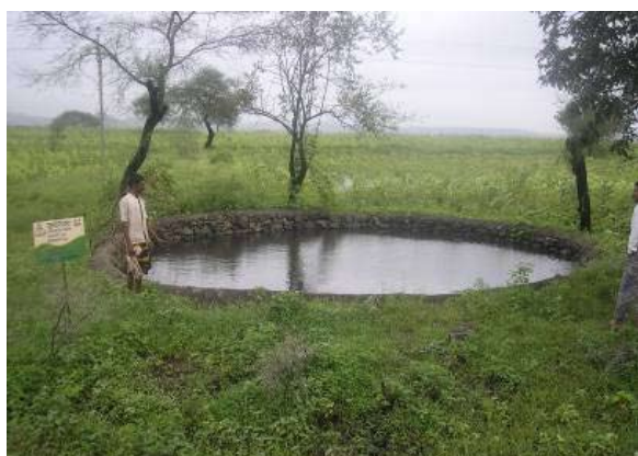
Dug wells recharged by in situ water harvesting
