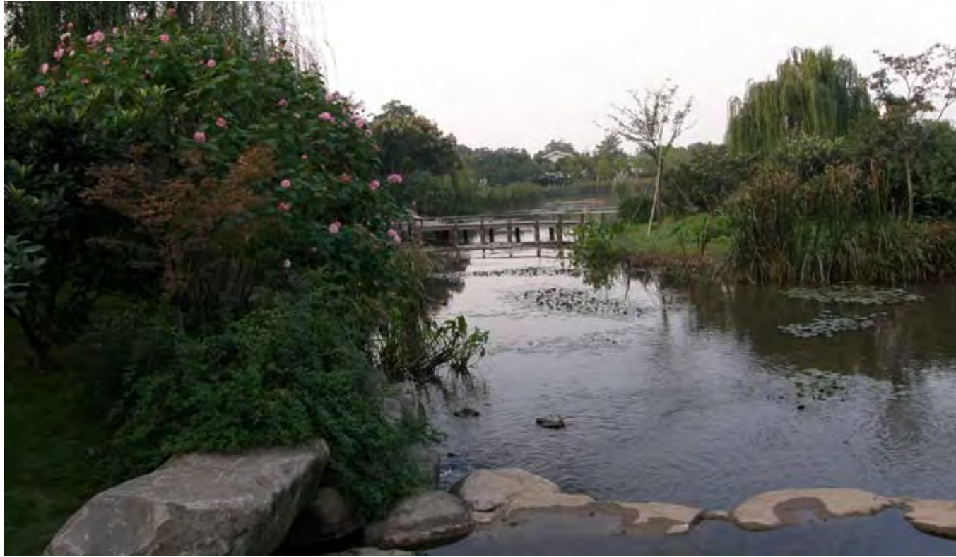
West Lake wastewater treatment by artificial wetland
