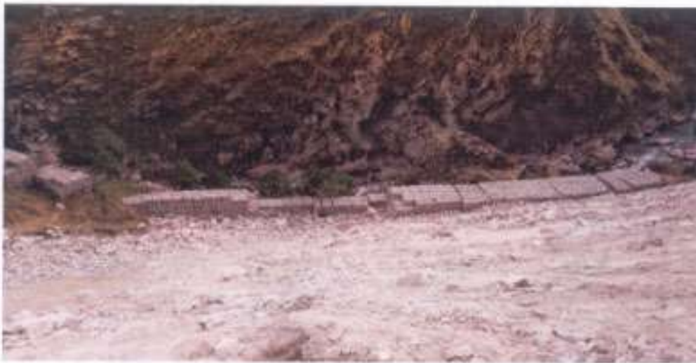
(Protection works provided for retaining the excavated material (muck))
