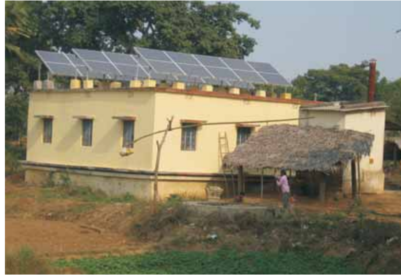
Power station at Kurawa Village, Jharkhand
