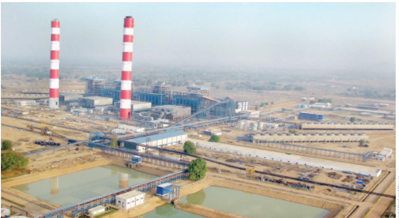
OP Jindal coal plant. Already the largest coal-fired IPP in India (1 000 MW), a brownfield expansion consisting of 4 x 600-MW units supplied by BHEL is underway. The site is also home to the largest private coal mine, coal washery, and covered coal conveyor belt in India.
