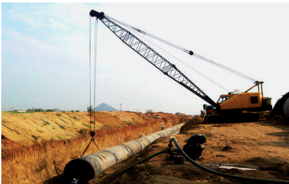
Mild steel pipeline being installed in Nagpur's water supply system
