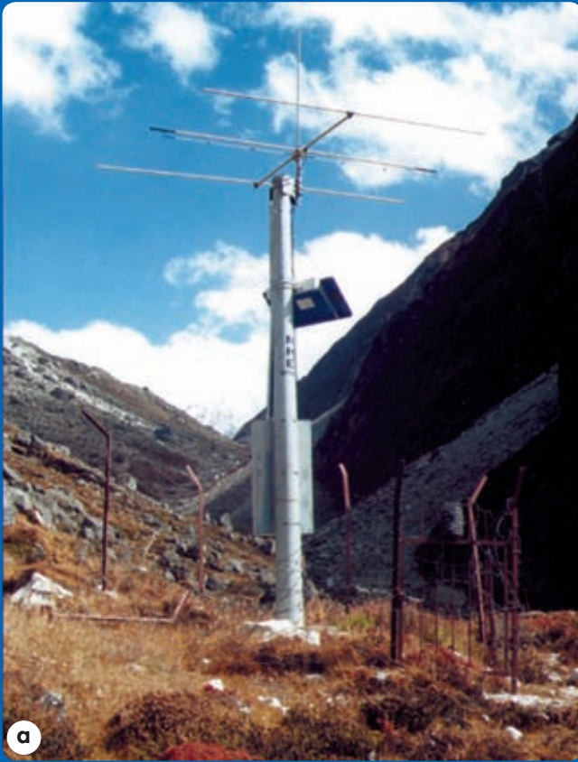
Figure 5: The Tsho Rolpa/Tamakoshi valley early warning system: a) Sangma Kharka transmitter station outside lake Tsho Rolpa receives signals from sensors and transmits to other remote warning stations; b) the warning and relay station Gongar village, comprising solar panel, battery, antenna and amplifier with siren; c) destroyed siren pole at Sigati village; d) damaged siren at Borle village
