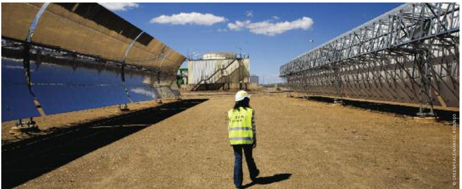
image A WORKER SURVEYS THE EQUIPMENT AT ANDASOL 1 SOLAR POWER STATION, WHICH IS EUROPE'S FIRST COMMERCIAL PARABOLIC TROUGH SOLAR POWER PLANT. ANDASOL 1 WILL SUPPLY UP TO 200,000 PEOPLE WITH CLIMATE-FRIENDLY ELECTRICITY AND SAVE ABOUT 149,000 TONS OF CARBON DIOXIDE PER YEAR COMPARED WITH A MODERN COAL POWER PLANT.
