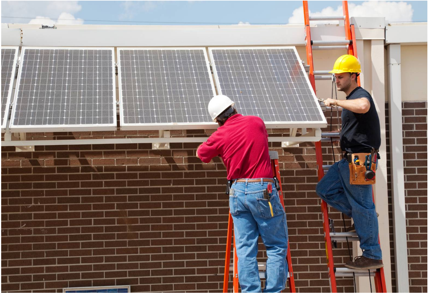
Men installing solar panels in Eastern Europe
