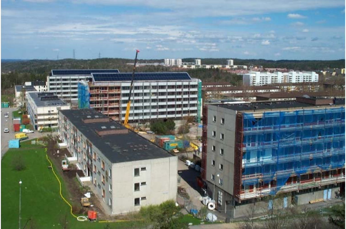
In Gardsten, Sweden, 1400 m 2 solar panels provide energy for some 500 flats
