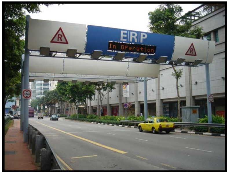
Figure 2: Electronic Road Pricing Gantry in Singapore (Copyright © 2005 Mailer Diablo) 1
