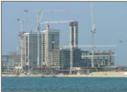
Large scale reclamation: man-made islands are being built in the shape of palm trees - Palm Jumeirah, Dubai UAE. Photo by: Peter Sale
