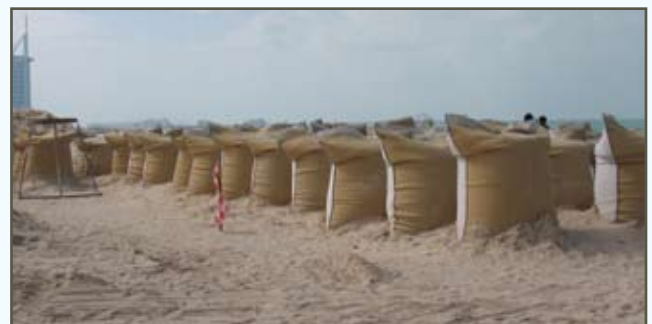
Large scale moderations to coastal areas can lead to beach erosion, as is the case here in Dubai, UAE. Good planning and comprehensive pre-construction environmental impact assessments that are properly implemented, can minimize these effects. Photo by: Hanneke Van Lavieren
