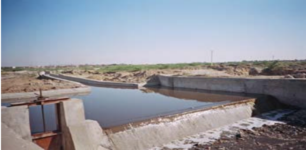
Figure: Gandhinagar drain being partially tapped into CETP III and rest bypassed
