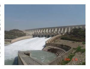
Since the reservoir capacity had reduced to 4.674 MAF from 5.88 MAF due to sediment deposition, raising of Mangla Dam by 30 ft. was taken in hand which has now completed. The Project will provide additional water storage of 2.88 MAF, increase water head by 30 ft and power generation of 644 GWh per annum and further flood alleviation.
