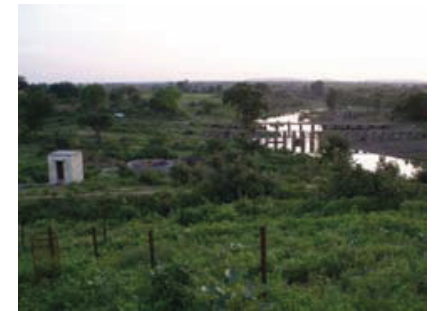
Figure 4. River bank infiltration well in Maharashtra
