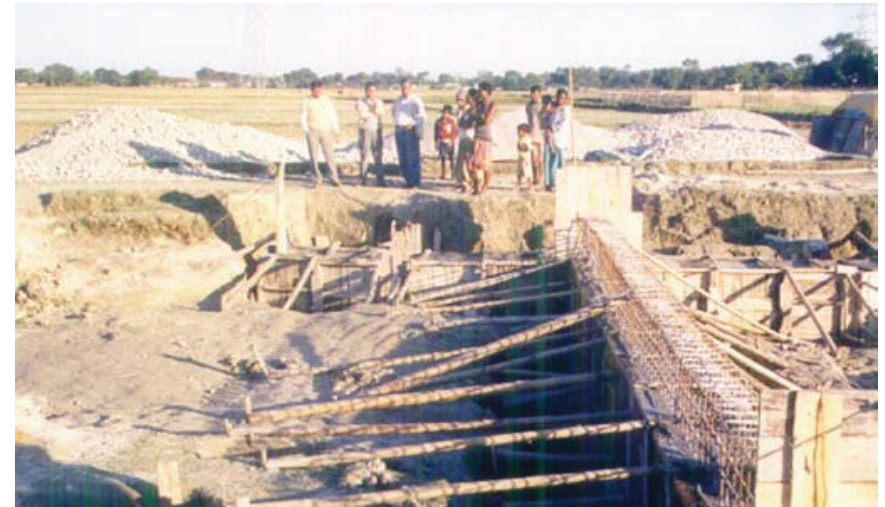
Figure 2. Constructing a gully plug to retain groundwater
