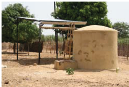
Figure 2. A hangar built by partner organization CCF as no appropriate roofs are available for roof water harvesting
