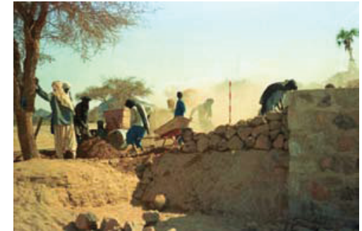
Figure 2: Construction of diversion works
