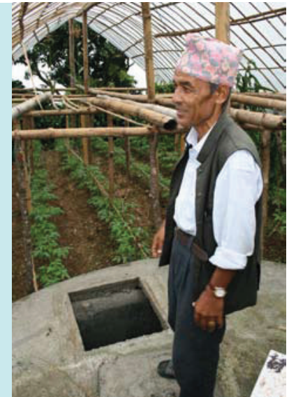
Figure 2. Owner of a rainwater harvesting tank and a biogas tank in Sarangkot, Palpa district, Nepal
