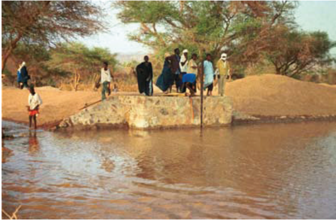
Figure 4: flood flow entering the infiltration basin
