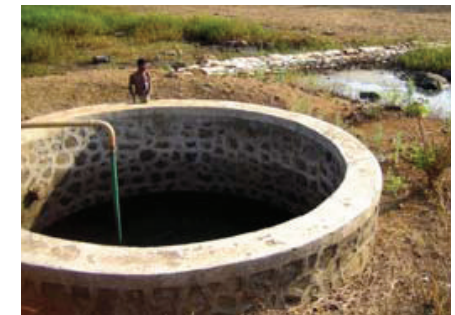
Figure 3. Open well adjacent to check weir in Vanuasi, India
