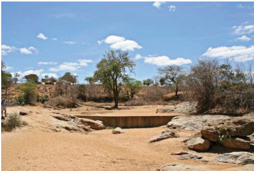
Figure 1. A typical sand storage dam during the dry season in the Kitui District
